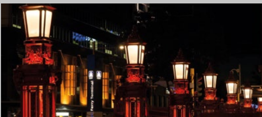
Red Fence Street lighting, NZ
